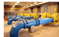
Pumping station site
