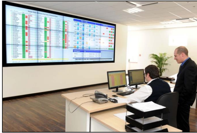
The newly refurbished WSC control Centre – 2012
